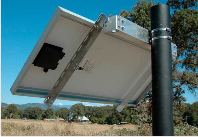
Figure 20: Solar panel mounting bracket
