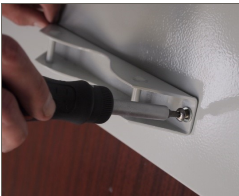
Figure 11: Attaching the banding bracket to the sign
