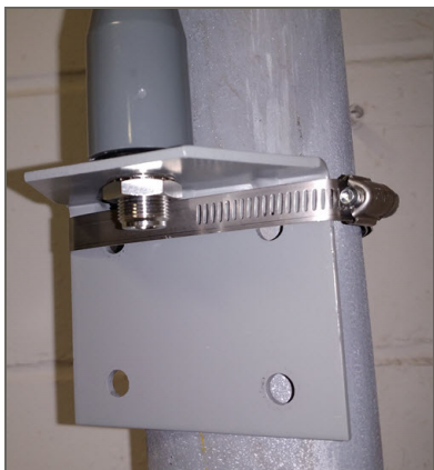
Figure 15: Antenna and bracket mounted with a banding strap
