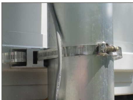
Figure 13: Sign Secured to a Pole with Banding Strap
